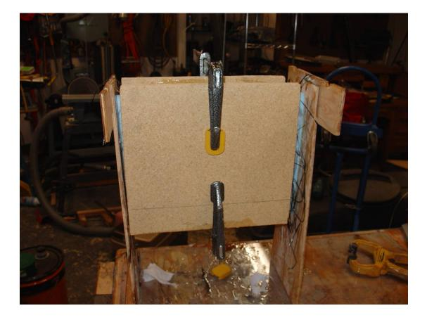
Use a hand saw to cut the cassette body from the stands. Clean it up by cutting the cassette ends square and end up with about a 9" long cassette. Use a carbide blade in your saw. Peel the breather cloth and peel ply off the outside of the cassette body.
